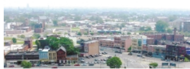
Adjacent to the Genesee Street block to the north on Ellicott Street is the Ellicott Lofts project with 34 loft spaces and 5,500 square feet of commercial use under construction. Another 60 living units are planned in phases over the next few years. (Source: The Urban Design Project)
