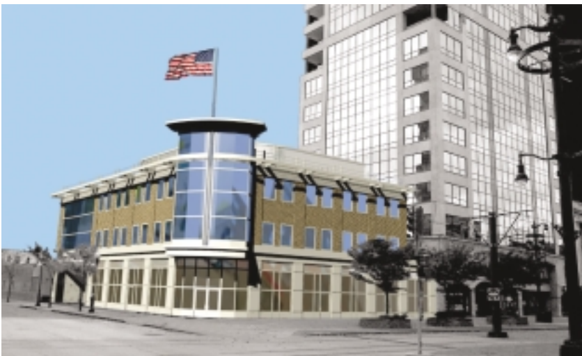
A new office building under construction at the corner of Main and Chippewa. (Source: City View Properties Inc.)
