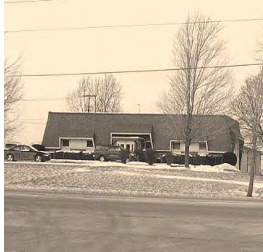
31. Existing parking lot in front
