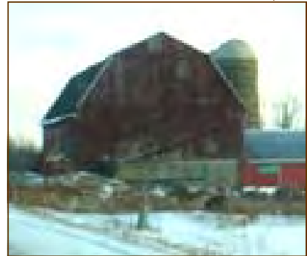
11. Local example of Gambrel roof style
