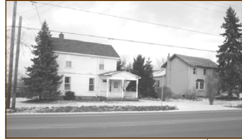
26. Existing condition showing direct access to corridor from individual parcels
