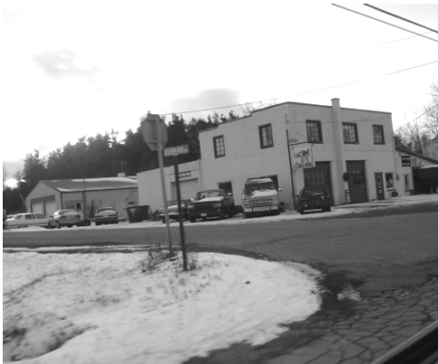
33. Existing corner lot building with open curb cut on both frontages
