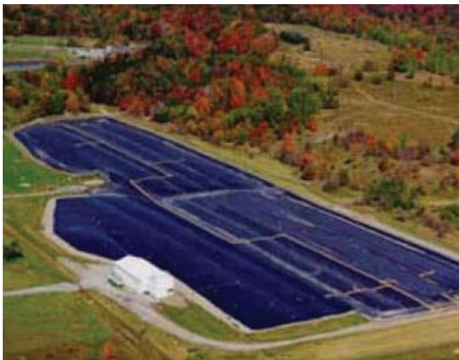
A birds-eye view of the SDA with a 15 acre geotextile cover. Source: Joanne Hameister
