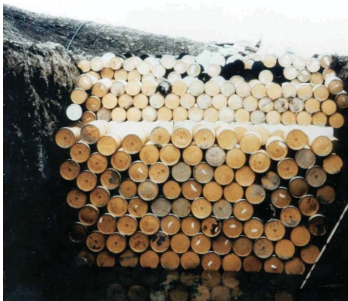
Waste was placed in plain dug, unlined, erosion-prone trenches. The DOE and NYSERDA want the waste to remain in these trenches, while the CWVNW wishes for the waste to be exhumed.
