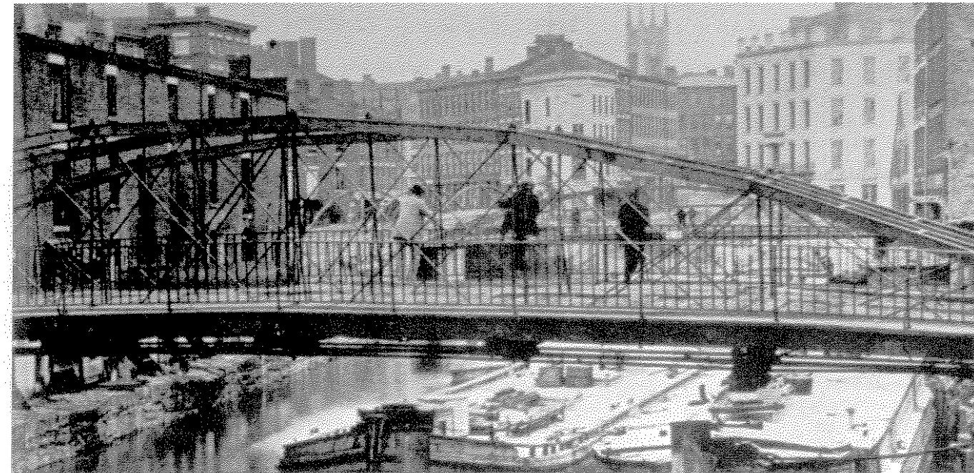
Arch Truss over the Commercial Slip, Circa 1870.
