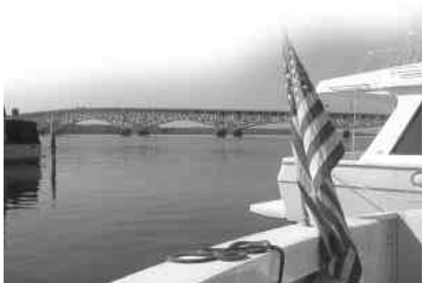
North Grand Island Bridge.
