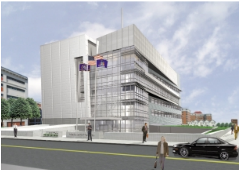
Artist's rendering of the new $33 million Erie County Public Safety Center. (Source: Image courtesy of Erie County and Cannon Design)
