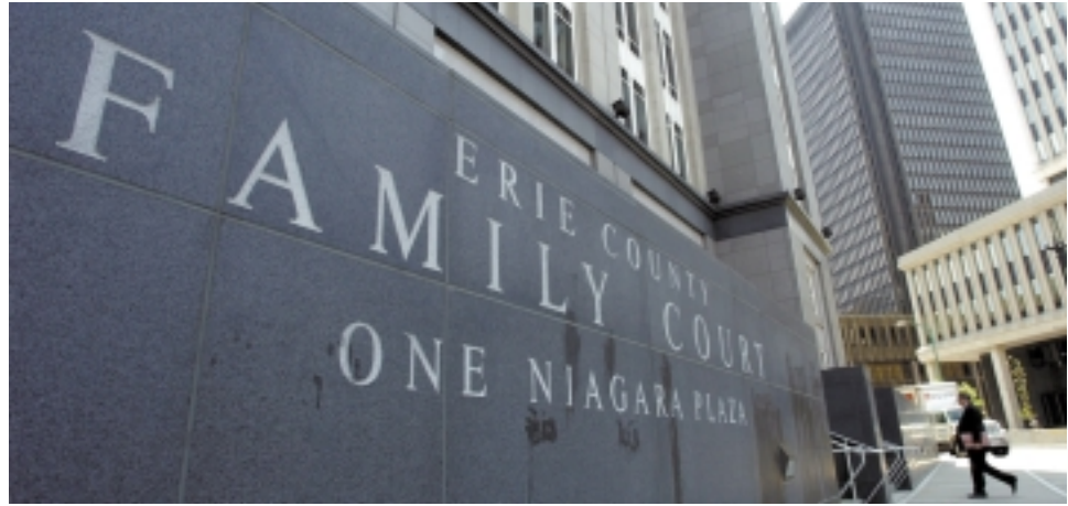
The newly constructed Erie County Family Court Building (Source: The Buffalo News/Robert Kirkham)
