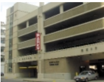
The Robert Adam Ramp on Washington Street is receiving additional levels to increase its total capacity. (Source: The Urban Design Project)
