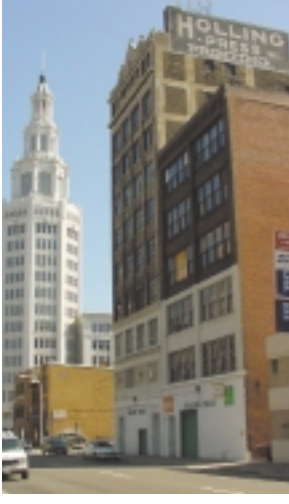
The Holling Press Building on Washington Street adds balance to the current market rate apartments with the addition of affordable units meeting the needs of Downtown workers with annual incomes below $35,000. (Source: The Urban Design Project)
