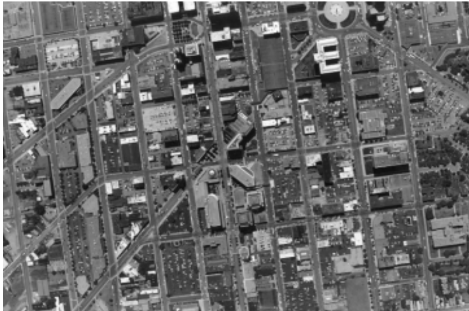
The and density of the Downtown core invites exploration of shared energy infrastructure including the potential for district heating. (Source: City of Buffalo)
