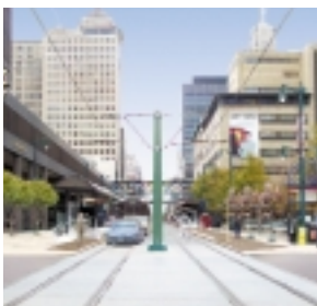
The preferred alternative to cars sharing Main Street is for cars to share the track bed. (Source: Buffalo Place Inc.)
