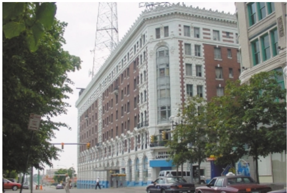
The Lafayette Hotel is a Local Landmark and is National Register Eligible. (Source: The Urban Design Project)
