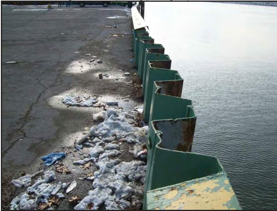
Photo 10 – Missing channel cap along parking lot portion of wall
