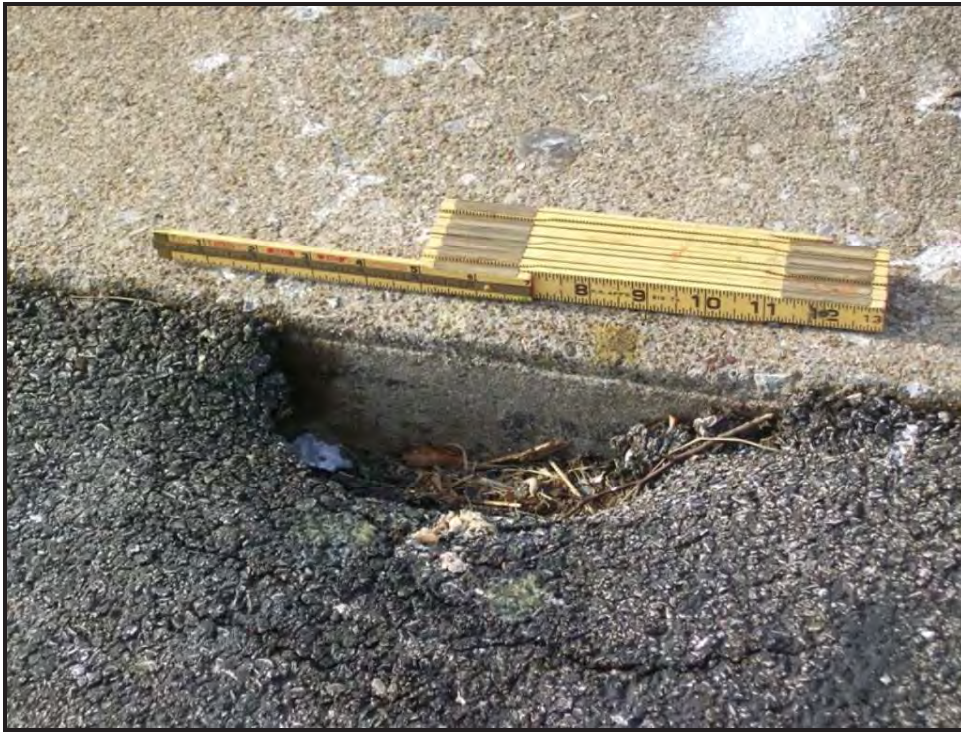
Photo 14 – Settlement in wall backfill
