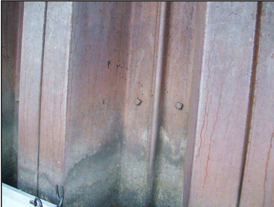
Photo 11 – Missing washer plates on whaler connection bolts
