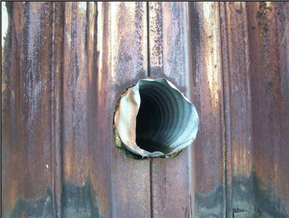
Photo 13 – Steel culvert penetration thru wall (Station 18+00)
