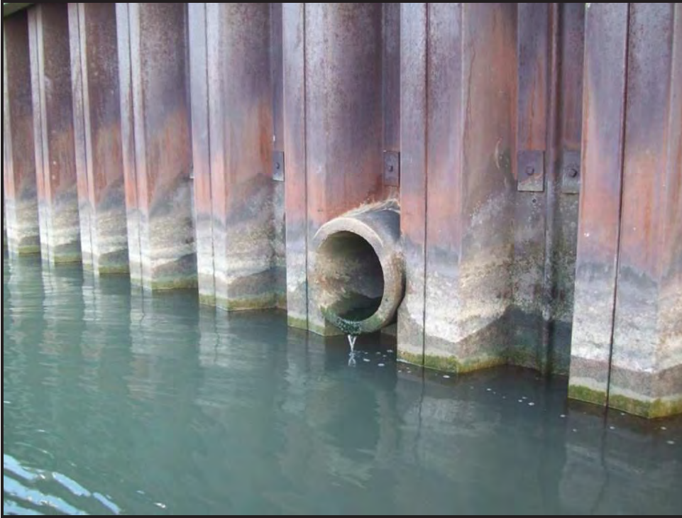
Photo 12 – Concrete culvert penetration thru wall (Stations 3+68, 8+00, & 12+20)
