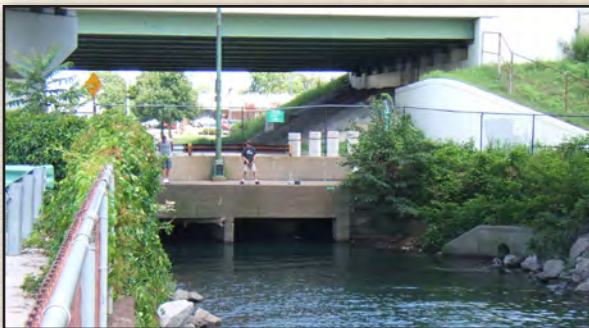
Cornelius Creek is daylighted through a box culvert that passes beneath the park entrance road, above.
