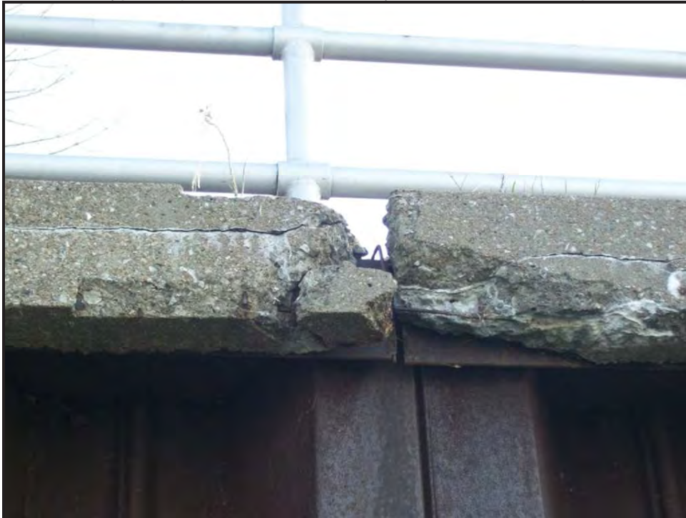
Photo 9 – Typical spall in concrete overlay on steel channel cap
