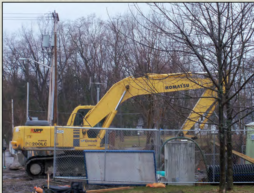
Work Progressing on the Town of Evans Waterline and Road Improvements - peter j. smith & company
