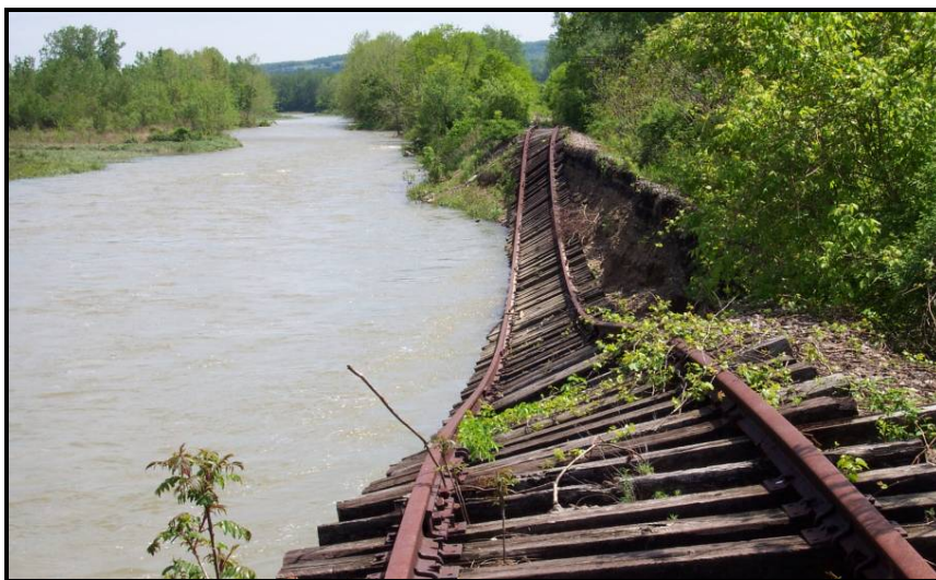
Figure 58 Southern Tier Extension Washout 2002
