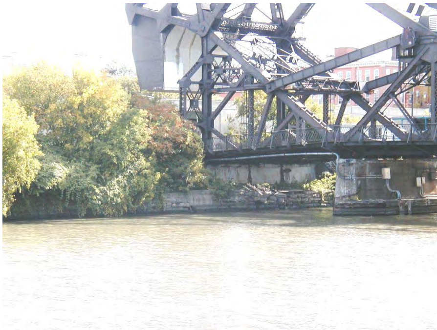
Stacked Stone Retaining Wall under W. Ferry Street Draw Bridge
