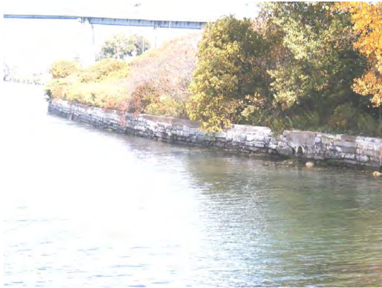
Stacked Stone Retaining Wall South of the Peace Bridge
