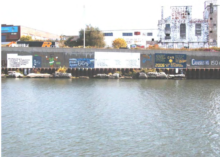
Stacked Stone Retaining Wall and Sheet Piling South of W. Ferry Street Draw Bridge. Also shows Concrete Retaining Wall for I-190 in this area.
