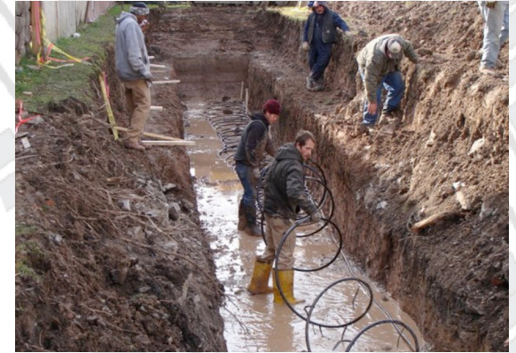
PUSH staff and trainees install a geothermal heating system for the NetZero House.
