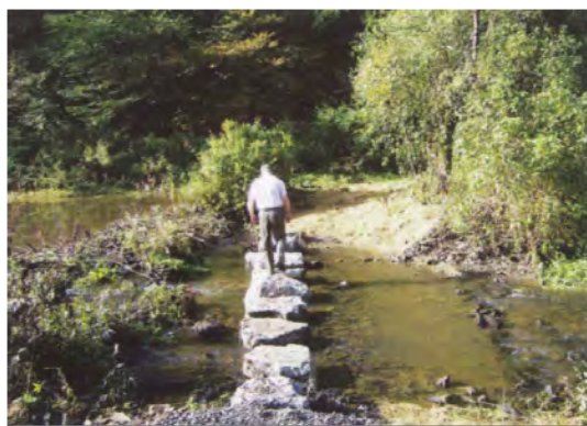
This section of the Finger Lakes Trail crosses the Cheningo Creek using large boulders in place of a traditional bridge. Taylor Valley State Forest, Cortland County
