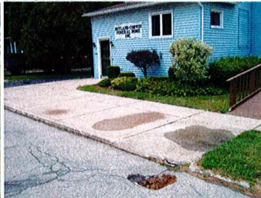
Pallister Avenue between Church and Coleman / Poorly situated CB in front of Funeral Home.
