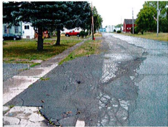
North side of Main Street near Pallister showing broken, uneven pavement sections, lack of curbing and insufficient drainage.
