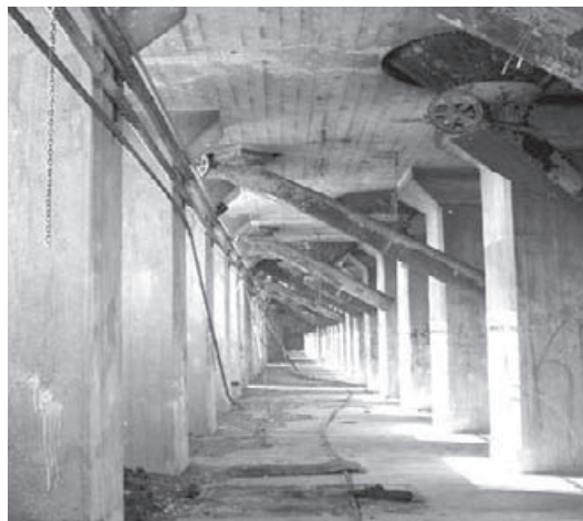
The Concrete Central elevator showing the raised basement, an invention of Harry R. Wait. (Photo by Lynda H. Schneekloth)
