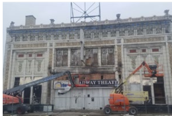
Broadway Theatre received support for building stabilization.
